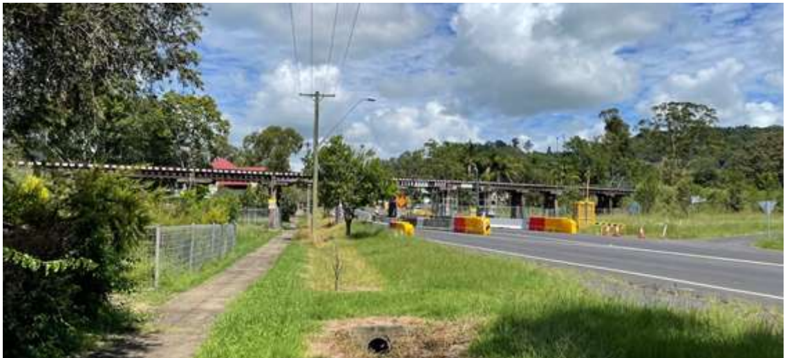
Figure 1.8 showing Terania Street underbridge looking west. Source TfNSW January 2024
