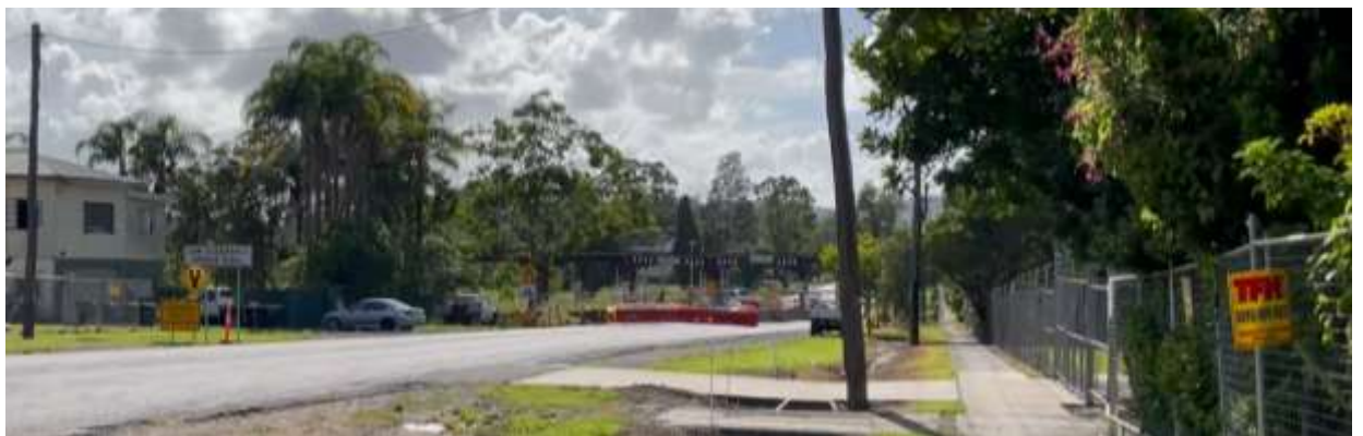
Figure 4.1 Photo of Terania Street underbridge taken at Tweed Street corner, showing a low lying single storey horizontal structure that is not highly visible along the street from any distance. (facing east). Source TfNSW February 2024
